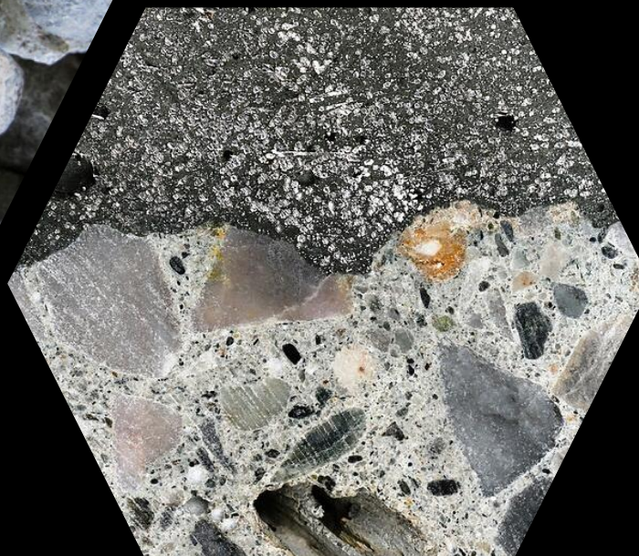
béton fibré ultra-performant UHPC
